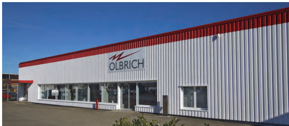
Innovationshalle in Goslar
